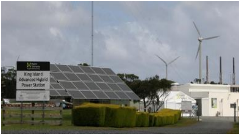
Hybrid Power Station
